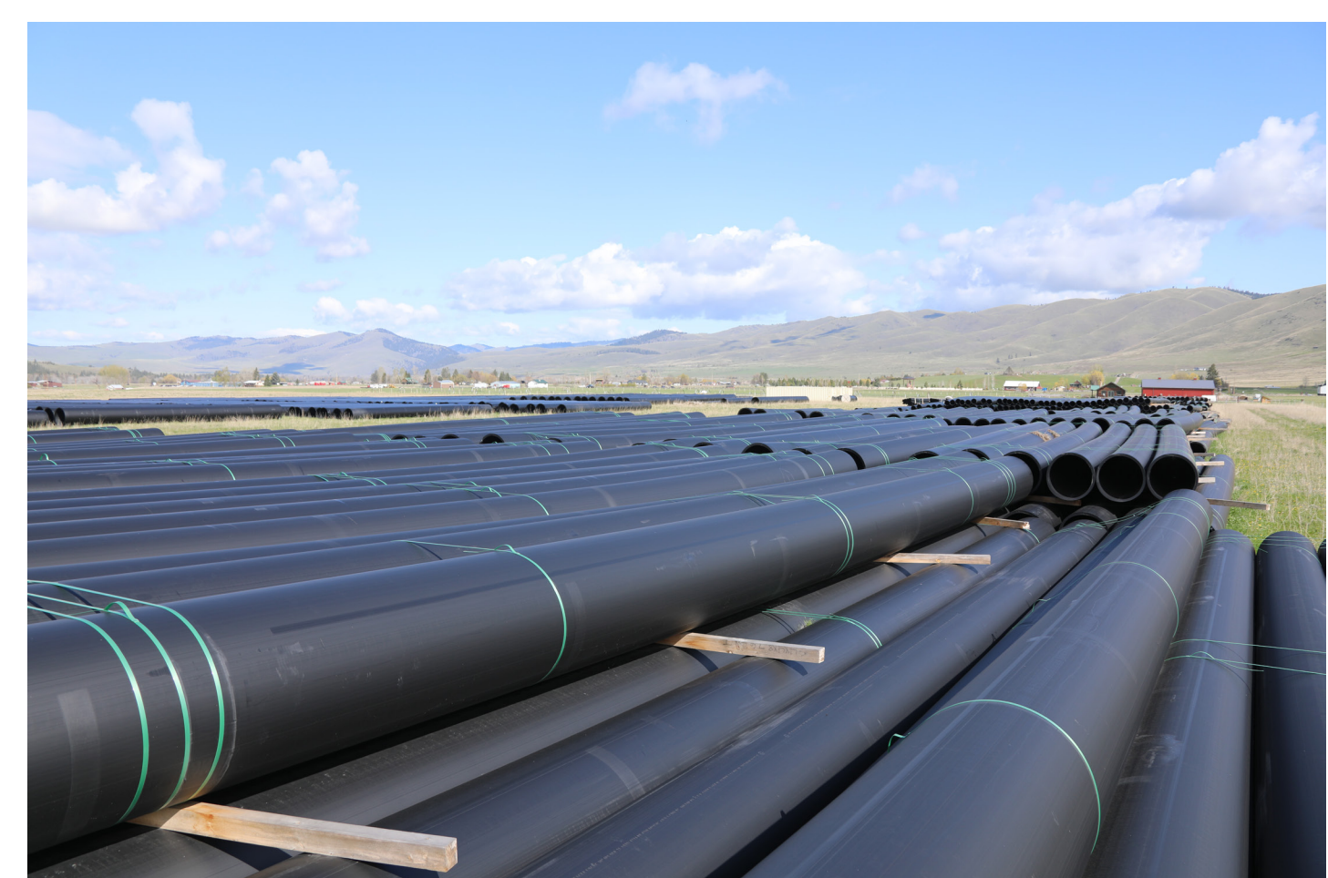
Large-diameter buried pipeline installed as part of approximately 18 miles of irrigation system upgrades in the Jocko Valley.
