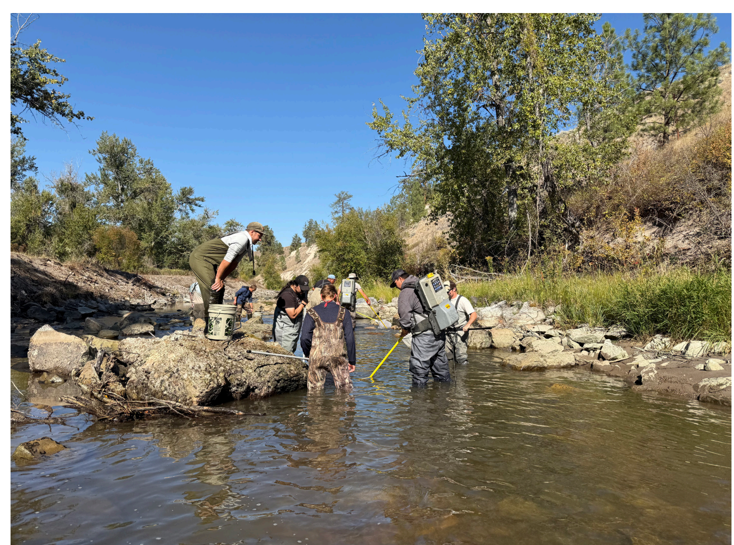
Fish rescue operations during fall 2025 helped protect native fish during active restoration work. Similar efforts are expected during future construction phases
