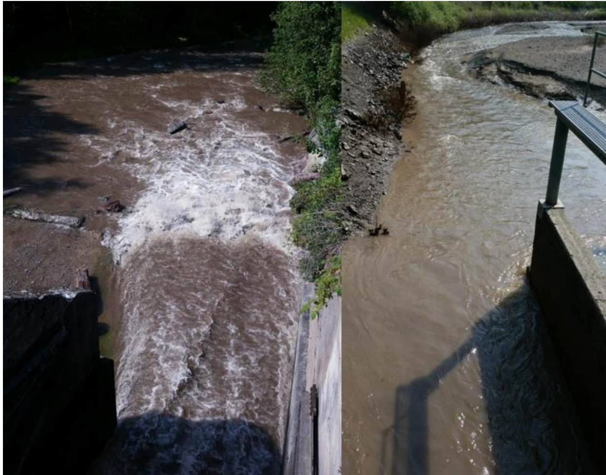
Figure 2: End-of-season sediment sluicing to pass accumulated sediment downstream of the Tabor Diversion.
